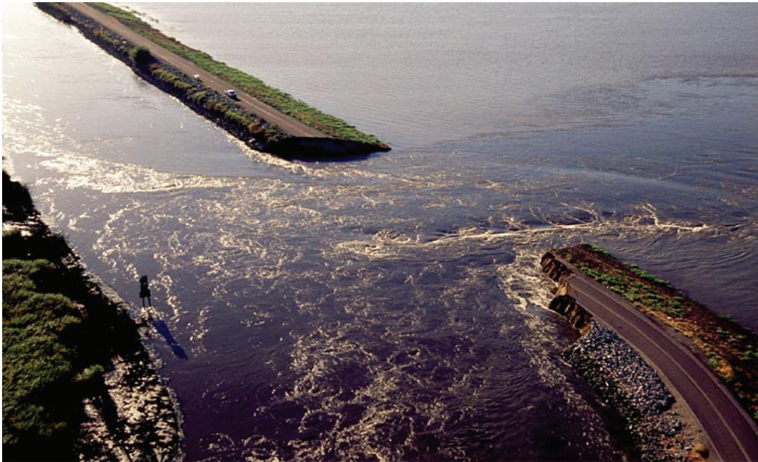
Figure 1.2 Water flowing into Upper Jones Tract from the Middle River after the levee break (photo)
